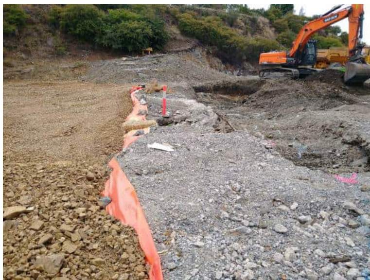
Plate 2 The Escarpment - Liner on the Western Boundary of the Telecommunications Cable
